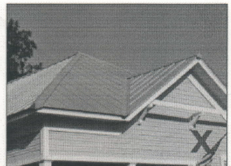
Do not use ridge caps with vents (left) or end caps (right).
